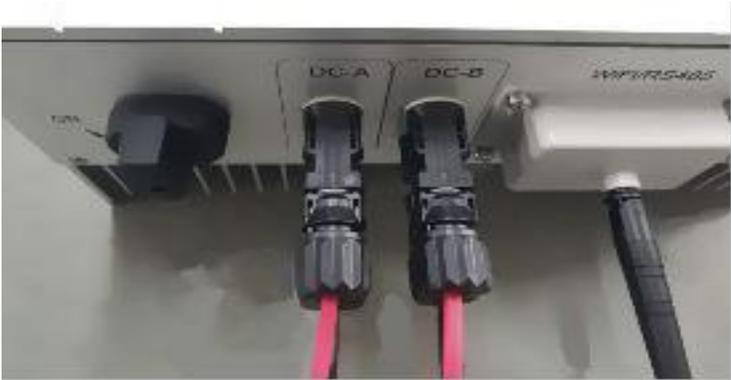
The inverter DC input is equipped with two groups(DC-A and DC-B) of connecting sockets for DC input , and each group contains two pairs of connecting sockets (DC+ and DC-). Make sure at least one pair of DC terminal in each group is connected with PV array in installation,and group A and B must be connected with two arrays separately but not with one array,see picture below.
